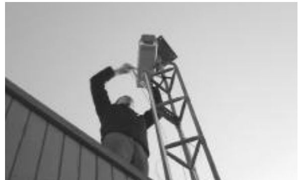
The Landcam being installed at the CLUI, Wendover.
